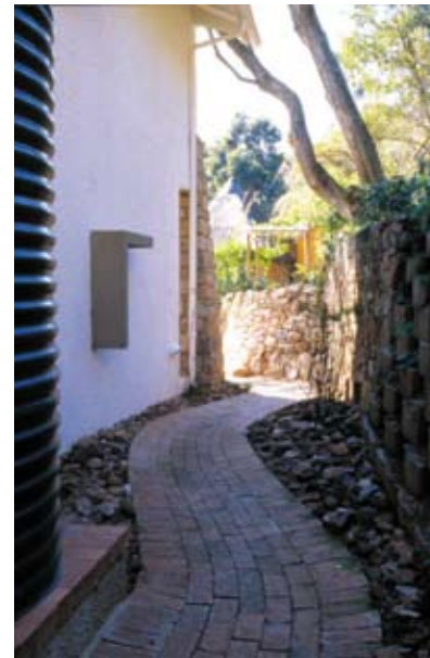
Water storage with landscaping used to absorb rainfall and a pathway profiled to take surface runoff to a reed bed
