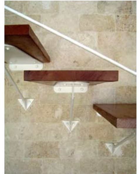
Rosewood stair treads on light steel supports
