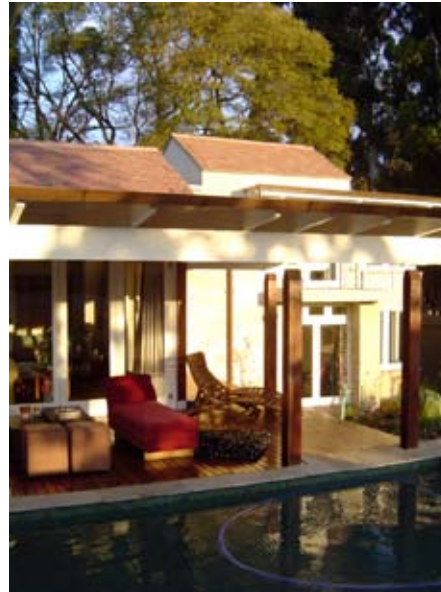
Copper gutters and natural timber posts
