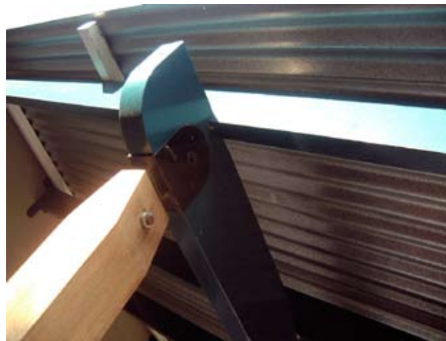
Wooden or steel column junctions
