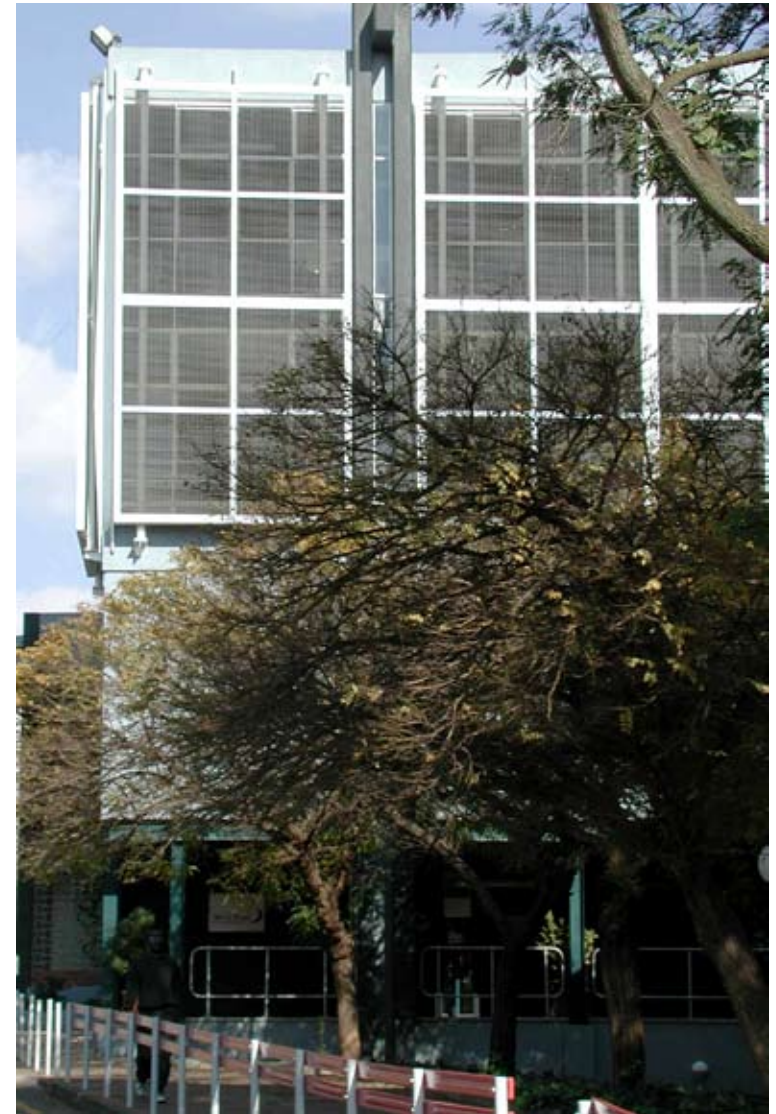
Filigree sun shading retrofitted to an uninhabitable building
