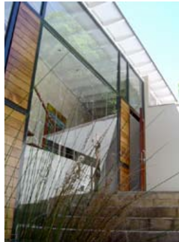
A south facing window wall to an entrance hall
