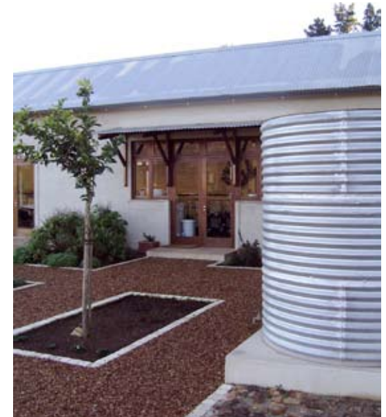
Water storage with landscaping used to absorb rainfall and a pathway profiled to take surface runoff to a reed bed
