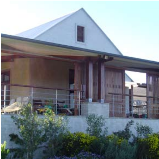
West facing verandah with sliding shutters for sun protection
