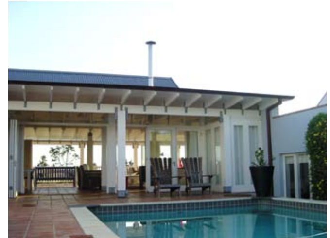
Folding doors that allow internal spaces to connect with the outside
